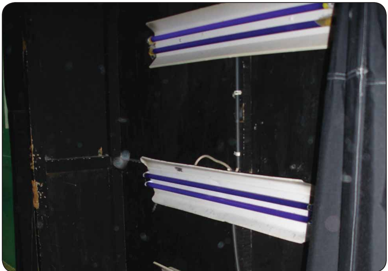
Figure 8 – Installation of Ultra Violet lights in the packing and inspection departments
